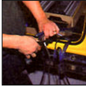
10 – From the fuse and ground distribution blocks, 8-gauge cables were wired in and cut to length so that they could be wired directly to their respective amplifiers. Lightning makes this gorgeous silver cable, one with a clear jacket and another with a translucent blue jacket; it complements any installation.
