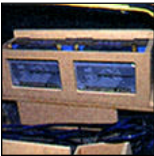
25 – A pair of Lightning Cells were also installed in the trunk. This endeavor started with a basic MDF box.
