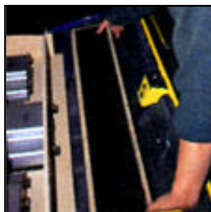
20 – With the caps out of the tray, it was positioned in the trunk and mounted for good. At that point the caps were dropped back into place and their brackets lined up with the holes that had just been drilled.
